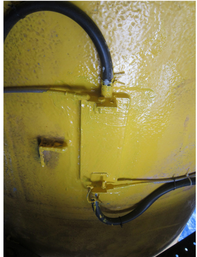
Fig. 9. The strain gauge on the surface of the pile.
